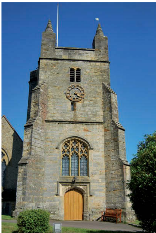
Fig. 3. Bolney tower, west face.
