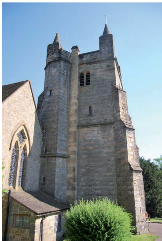
Fig. 2. Bolney tower, south face.
